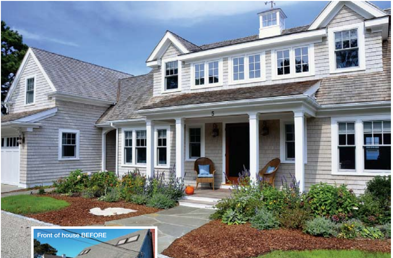
A Nantucket dormer — two gable dormers connected by a shed dormer — transforms the front of the house and adds space upstairs.
